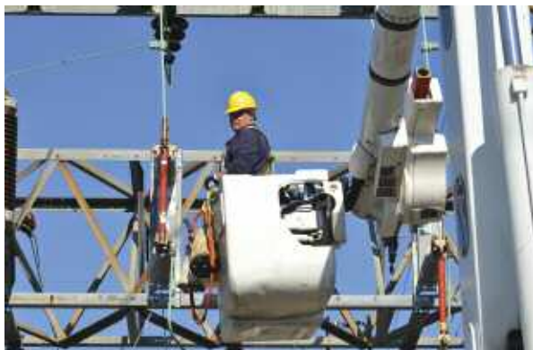
AT LEFT: Journeyman Lineman Bill Bogel, from the Martinsburg District, completes installation of new expulsion fuses at the Frankstown Substation as part of a day-long improvement project. The substation is located along Scotch Valley Road, right.
