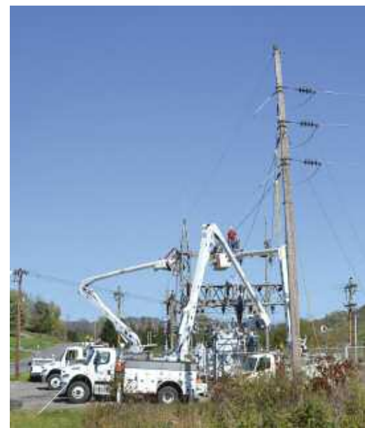
AT LEFT: Journeyman Lineman Bill Bogel, from the Martinsburg District, completes installation of new expulsion fuses at the Frankstown Substation as part of a day-long improvement project. The substation is located along Scotch Valley Road, right.
