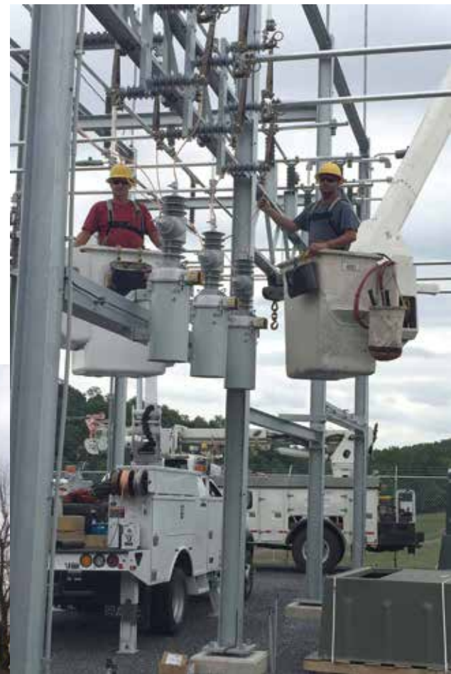
ABOVE: Crew Leader Kenny Sipes, left, and Journeyman Lineman Jonathan Shields place expulsion fuse hangers at the new Reeds Gap Substation in August.
