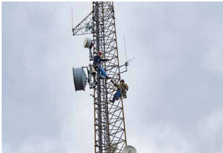
FROM THE LEFT: Dave Love and business partner Jerry Cox hang from Valley Rural's Loop Mountain tower next to the antenna that provides amateur radio for ham operators.
