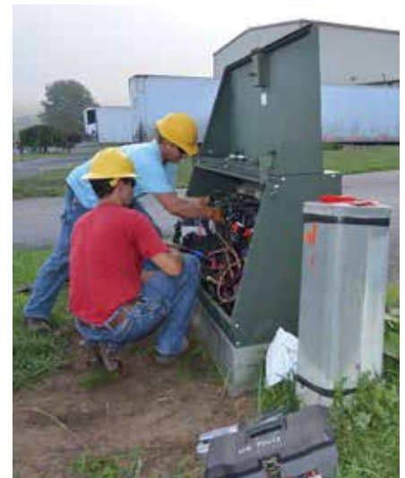
BELOW: Fourth Class Lineman Trevor Eichelberger (kneeling) and Journeyman Lineman Ryan Dodson connect service inside a cabinet near Shirley's Cookies.
