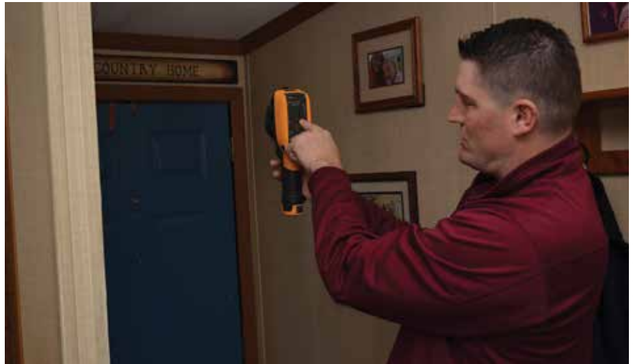
ENERGY AUDIT: Valley REC Energy Specialist Travis Kuhstos uses a thermal camera to see areas where air movement is flowing in and out of Carol and Jeff Sipes' home in McVeyton, Pa.
