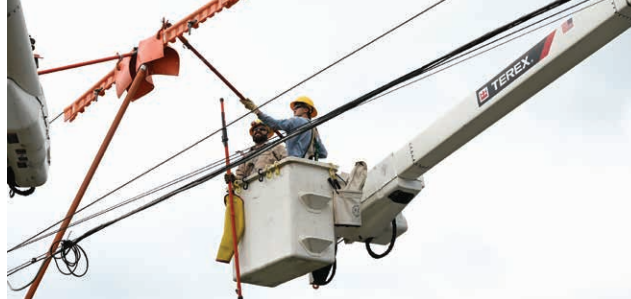
COVERING UP: Valley Rural Electric Cooperative Apprentice Lineman Carter Zerbe places protective plastic covers on a live line in Union Township, Huntingdon County.
