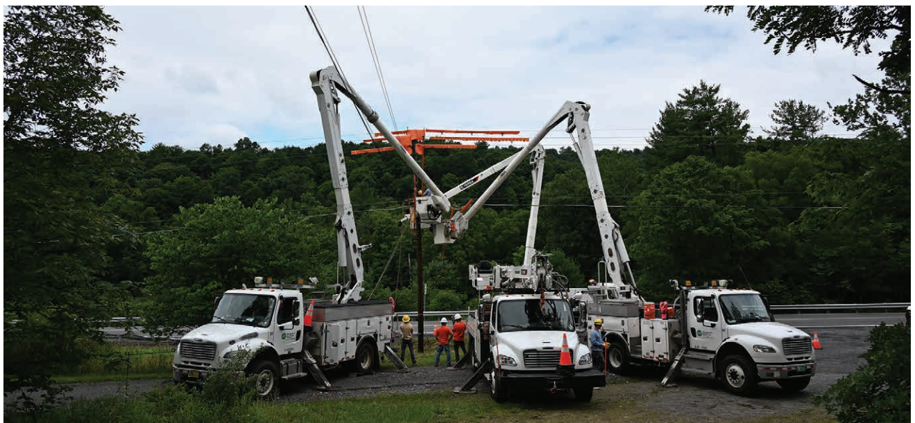
TRUCK TRIO: The simultaneous use of several aerial lifts is a hallmark of the annual on-the-job training at Valley Rural Electric Cooperative. Lineworkers can complete a pole replacement or other work while lines remain energized.
