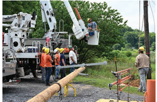
LIVE WIRES: PREA Job Training & Safety Program Instructor Ken Musick, center (in white shirt), and Valley Rural Electric Cooperative lineworkers review a pole-replacement job conducted in July in Union Township. During the project, the lines remained energized.
