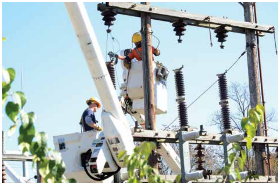
ABOVE: Journeyman Lineman Seth Glover, in the bucket at left, and First-Class Lineman Eric Yingling dismantle a portion of the wooden Atkinson Mills substation, which dates back to the 1950s.
