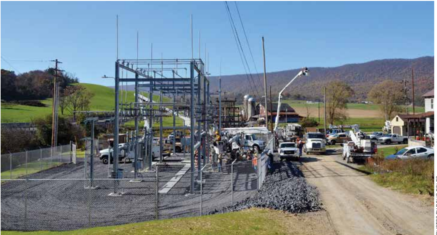
NEW SUBSTATION: Before energizing the new Atkinson Mills substation along Route 22 in Wayne Township, Mifflin County, Valley REC crews do some prep work at the site in early November. The new metal structure replaces the aging wood substation, which can be seen in the background.
