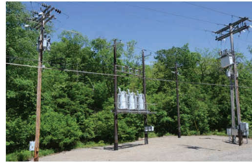
NEW POLES: Above – Three ductile iron poles are located at Valley Rural Electric Cooperative's (REC) Little Valley substation. Below – Valley REC Coordination Engineer Eric Henchey inspects regulator controls mounted to one of the ductile iron poles. The poles have a 70-year life span.
