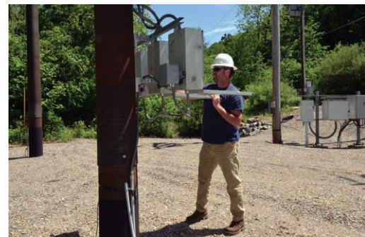
NEW POLES: Above – Three ductile iron poles are located at Valley Rural Electric Cooperative's (REC) Little Valley substation. Below – Valley REC Coordination Engineer Eric Henchey inspects regulator controls mounted to one of the ductile iron poles. The poles have a 70-year life span.
