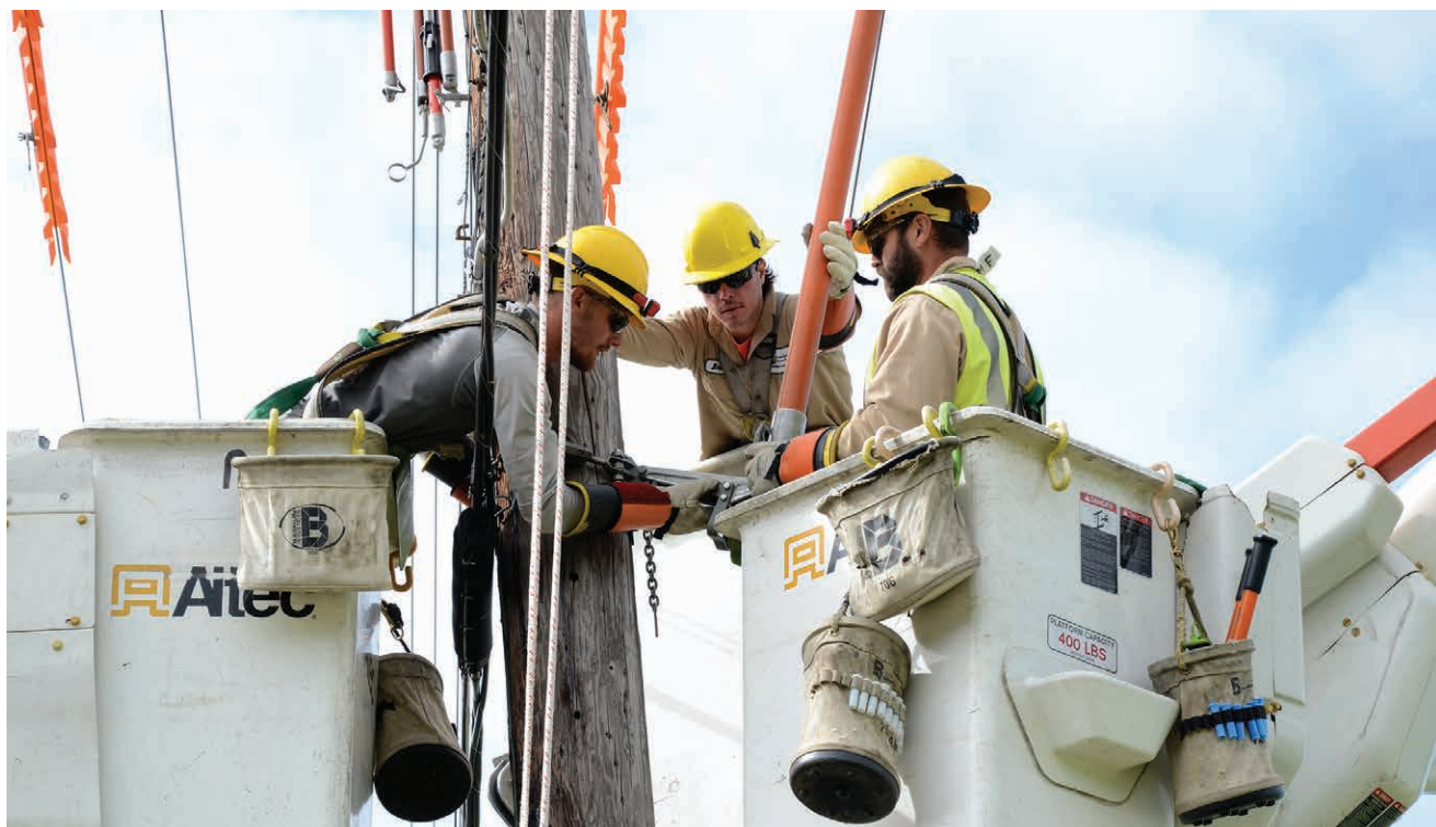
WORKING TOGETHER: From left, Valley Rural Electric Cooperative linemen Owen Winter, Bruce Perow and Matt Fish secure a fiberglass throw-out arm to a pole top. The work was done during annual on-the-job energized line training Sept. 10 in Greenfield Township, Blair County.
